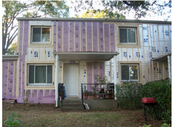
Block home with insulation, prior to siding installation. Staff photo.
